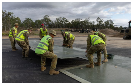
↑ Aviators from 65ABRS with counterparts from the Royal Canadian and US Air Forces prepare sections of fibreglass re-enforced panels to repair craters in an airstrip at Townsville Field Training Area.
